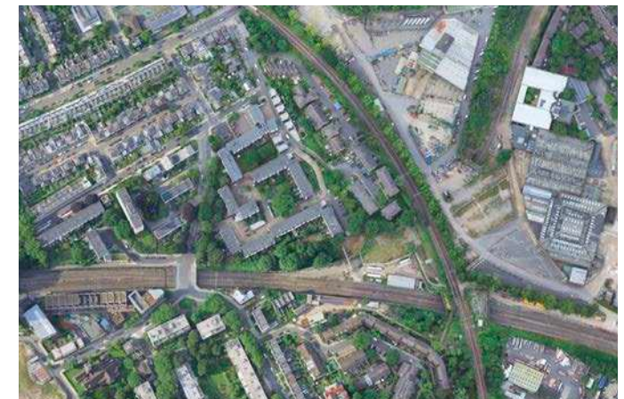
Aerial view after
