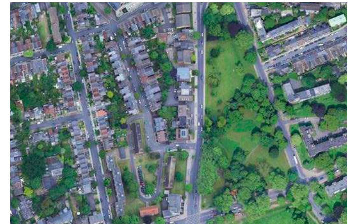
Aerial view after
