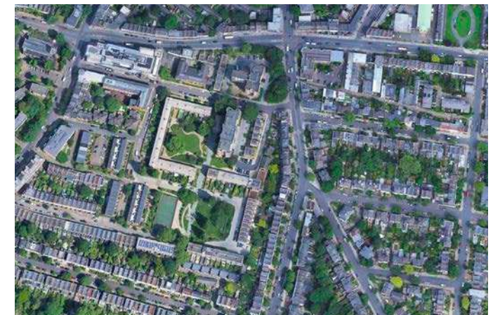
Aerial view after
