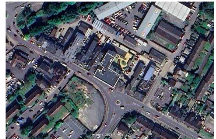
Aerial view after
