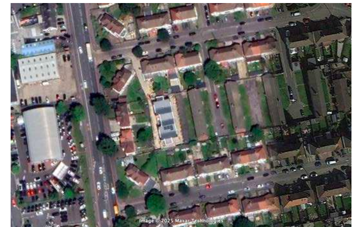
Aerial view after
