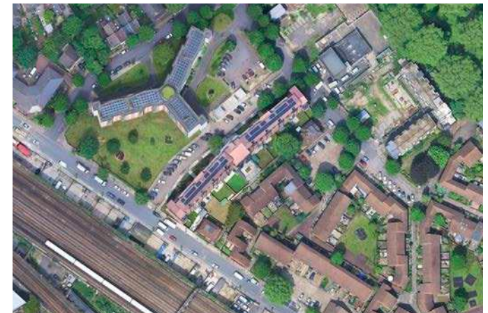
Aerial view after
