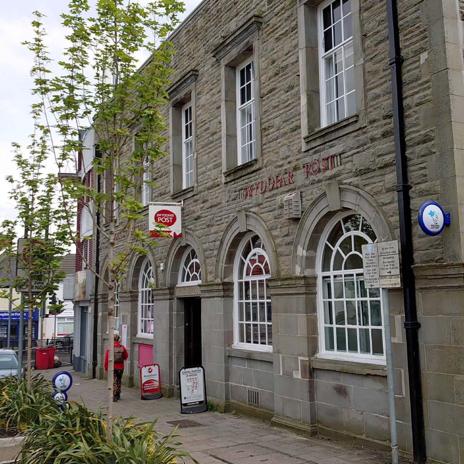
Morryston Post Office, with converted upper floors for housing and green roof. Complemented by the greening project in the public realm.
