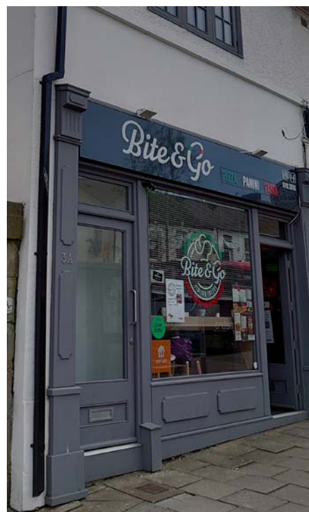
Shopfront improvement at 3 Woodfield Street, funded by WG Placemaking grant.
