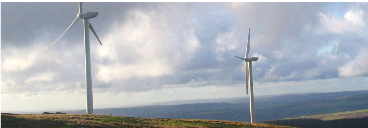
Ffynnon Oer Windfarm Access, UK © Arup
