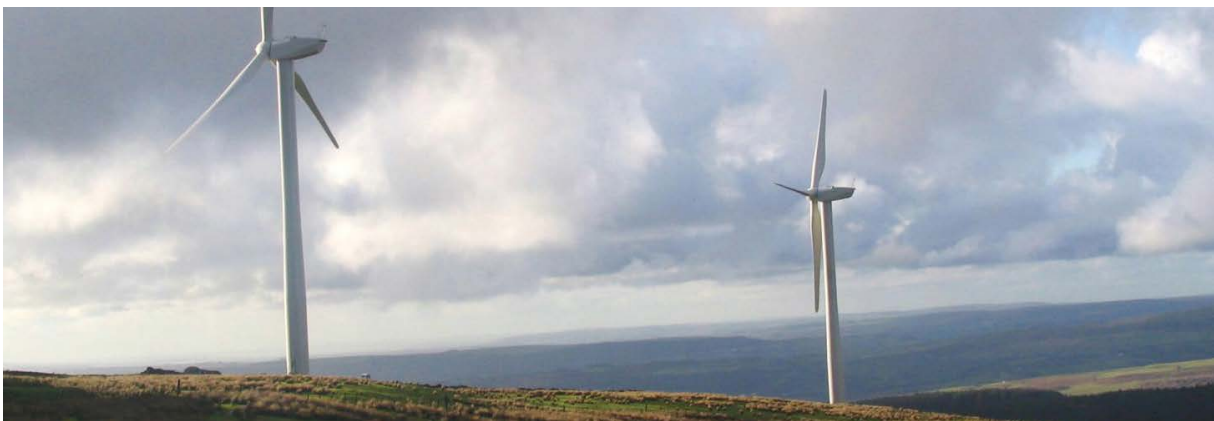
Ffynnon Oer Windfarm Access, UK © Arup
