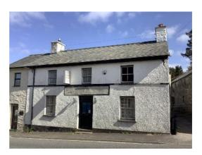
The current proposal sets out changes to the existing renovation. The intention is to remove roughcast sand and cement render on the front elevation and side wall and repoint using lime mortar with white lime wash to finish, with the objective of remedying the damp problems and allow the historic walls to 'function as originally designed using traditional lime mortar and lime wash'.
