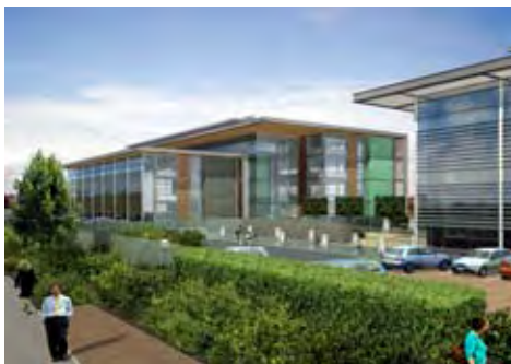
Case Study 14: Welsh Assembly Government and Ceredigion County Council Buildings, Aberystwyth. This view showed the Council Building in the foreground and the Assembly building behind, with the central space that they should share divided by a glazed screen. The full height atria provided a single central axis through both buildings and assisted natural ventilation.
